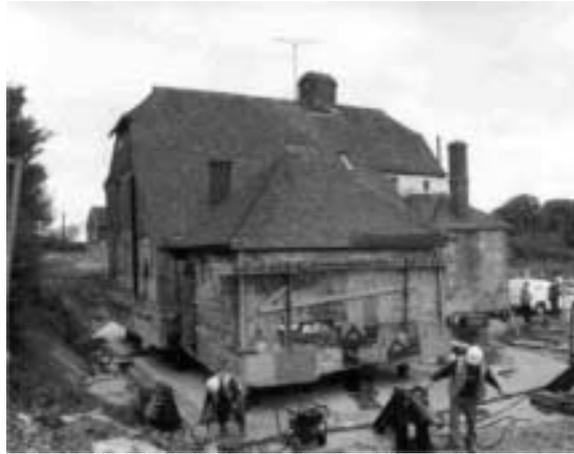
**Figure 1** CTRL UK—relocating Bridge House, 7 July 2000. Photograph courtesy of Abbey Pynford.
