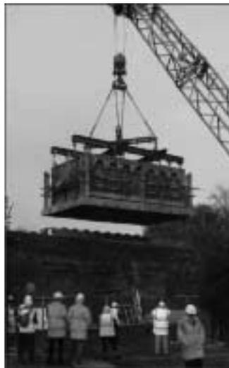
**Figure 4** CTRL UK—a section of the Waterpoint being lowered into its new position, November 2001. Photograph courtesy of the Architectural Heritage Fund.
